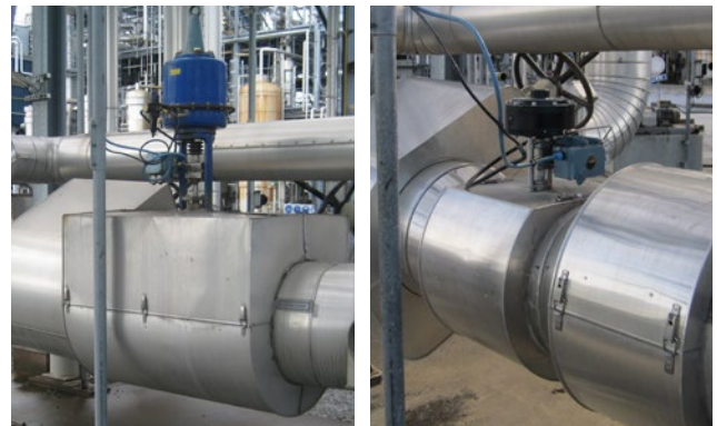
Before and after – Sliding gate valve DN250 in operation in the steam filter station at EVAL Europe N.V. in Antwerp.
