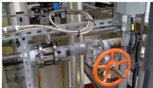
Fig. 6 The new sliding gate valve with 8049 positioner.
